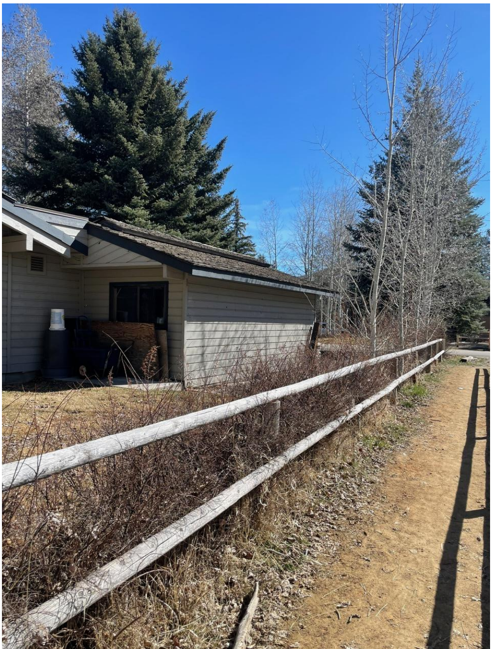
RIVER ACCESS EASEMENT VIEW OF GARAGE
