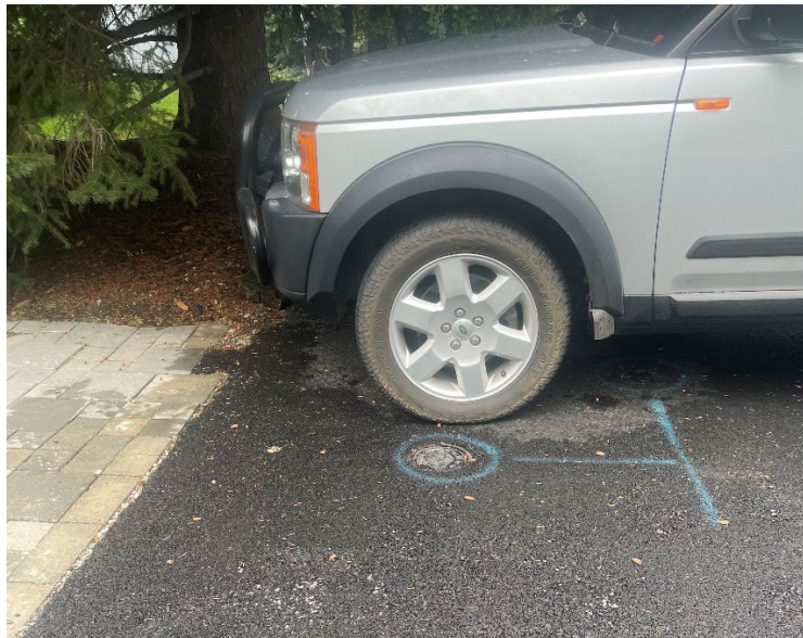
Figure 1 – Water line @ Driveway
