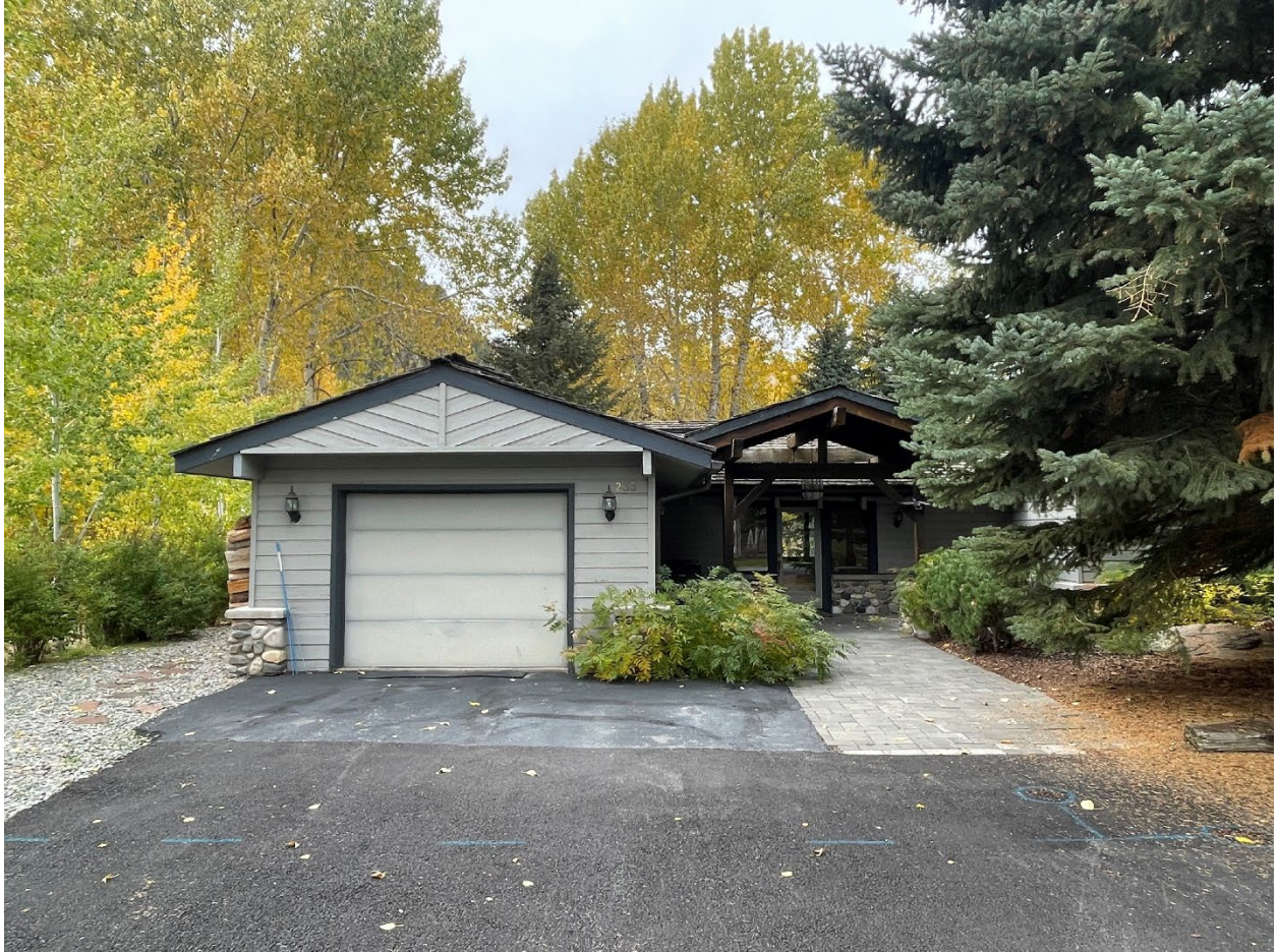
C. Existing Garage and Driveway
