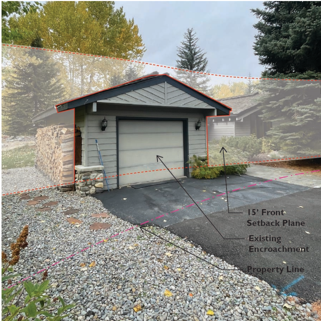
D. Existing Garage Encroachment into Front Yard Setback
