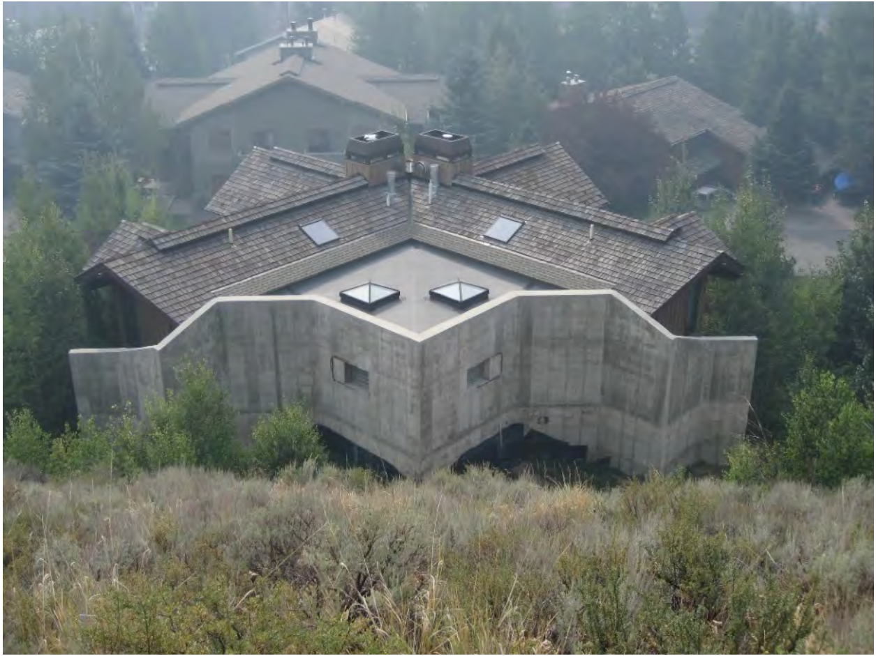
392 & 394 Sage Rd Avalanche wall integrated with building. Sits on massive footing with 2' deep keyway extending below footing to resist forward displacement.
