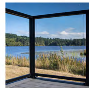
MAT 9 - Glass handrail with steel posts
