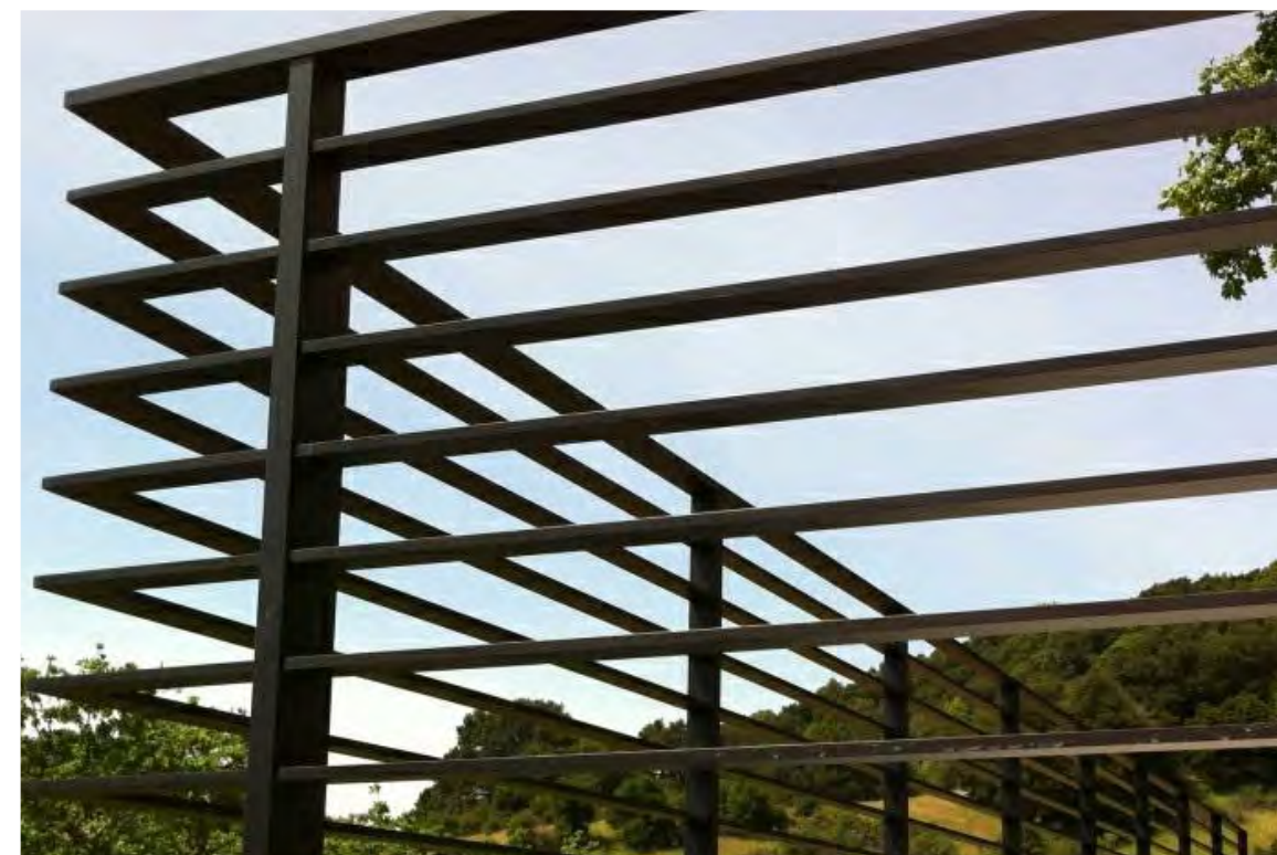
GUARDRAIL 1 (GR-1): BLACK STEEL BAR
