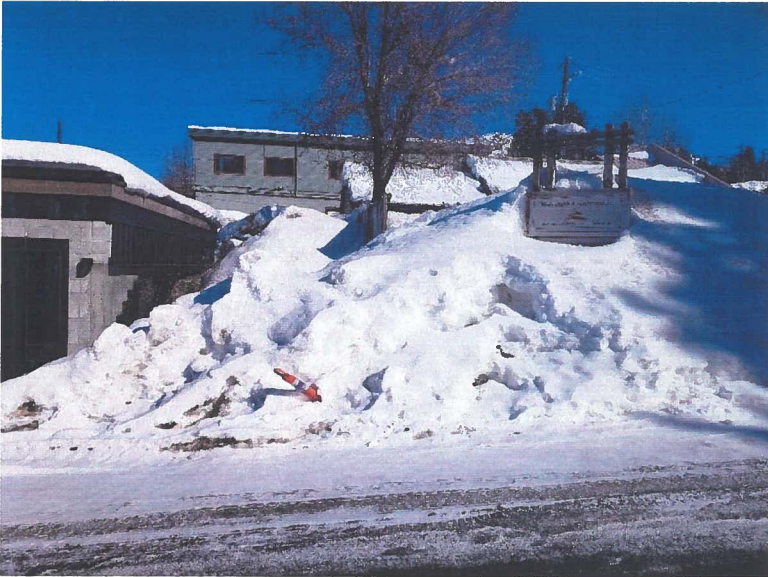
2 - Existing Site Conditions - Lot 3 existing grade at base of wooden sign. Grade in between sing and building is 3' lower than pavers.
