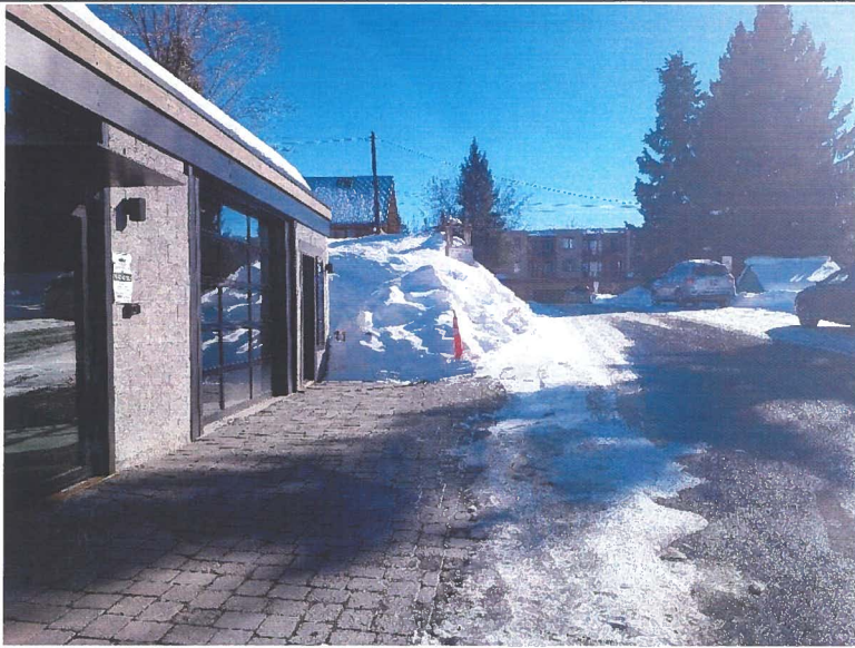
1 - Existing Site Conditions - Lot 3 existing grade at base of wooden sign. Grade in between sing and pavers is 3' lower than pavers.
