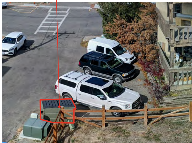
EXISTING CONDITIONS AT AREA OF CONCERN
