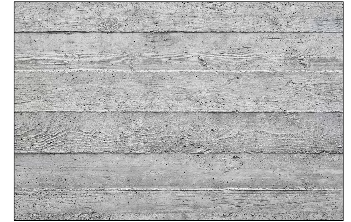
EXTERIOR FINISH 9 (EF-9): EXTERIOR CAST-IN PLACE BOARD-FORMED CONCRETE RETAINING WALL
