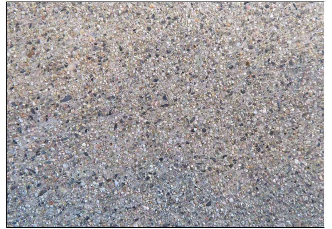
EXTERIOR FINISH 7 (EF-7): EXTERIOR CAST-IN-PLACE CONCRETE SLAB; ACID ETCHED CONCRETE WITH LIGHTLY EXPOSED AGGREGATE
