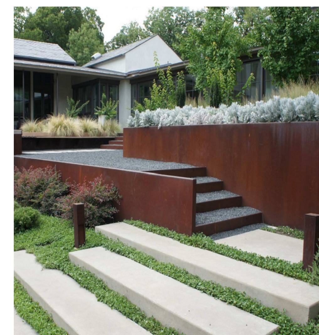
CONCRETE W/ STEEL PLANTERS AS RETAINING WALLS
