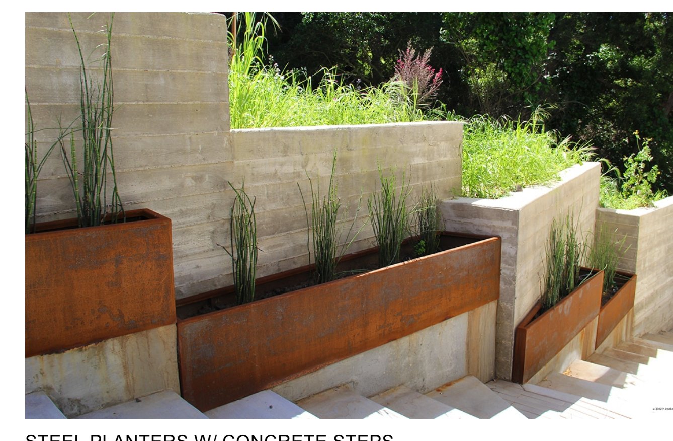
STEEL PLANTERS W/ CONCRETE STEPS
