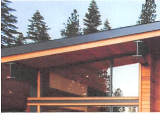
Fascia – Metal and Wood Fascia
