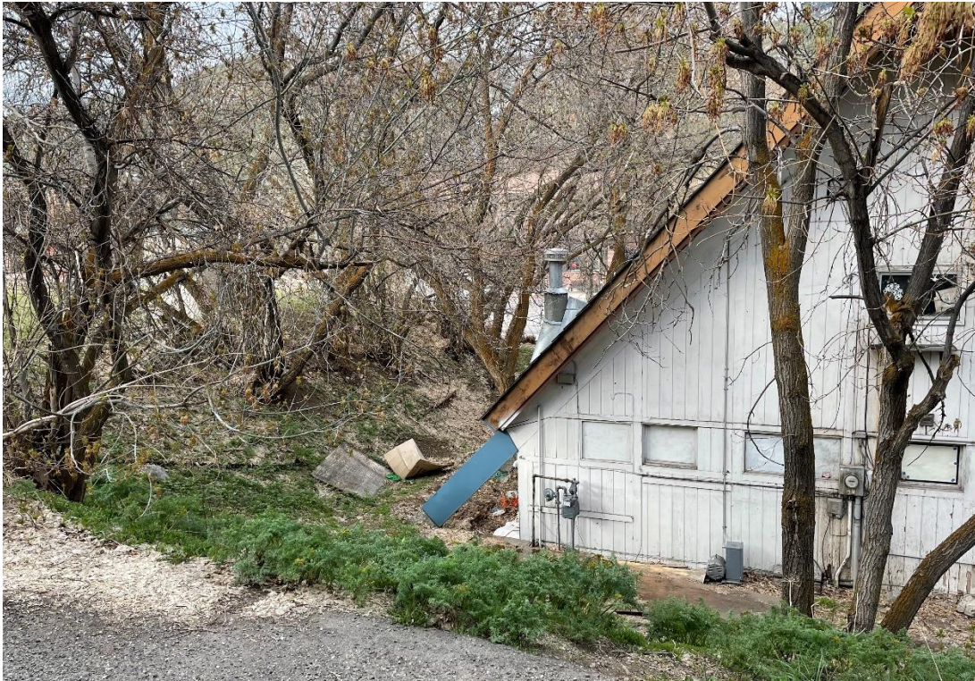
3. Back of Building
