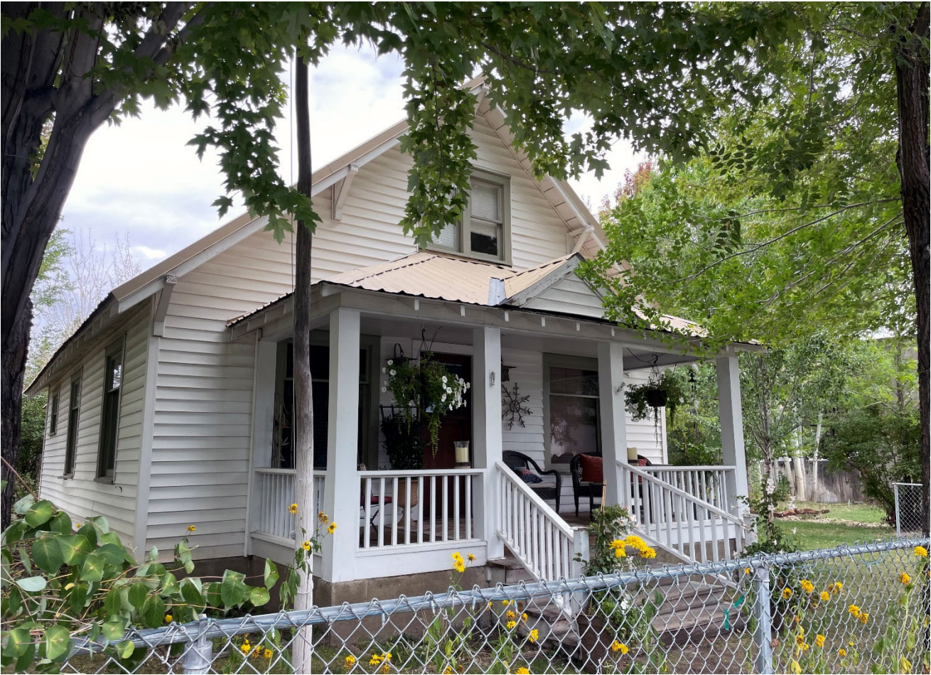
Photo A: Front Porch, Northwest side
