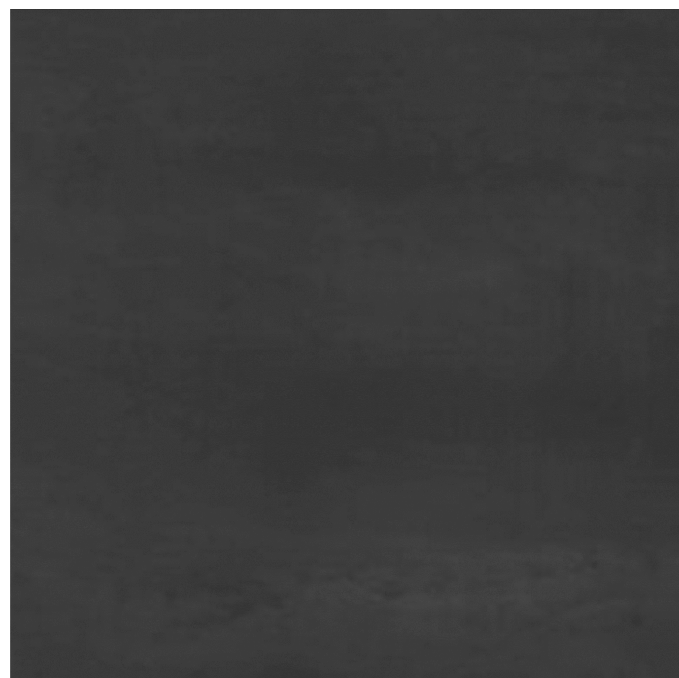
FINISHED GREY METAL ROOF
