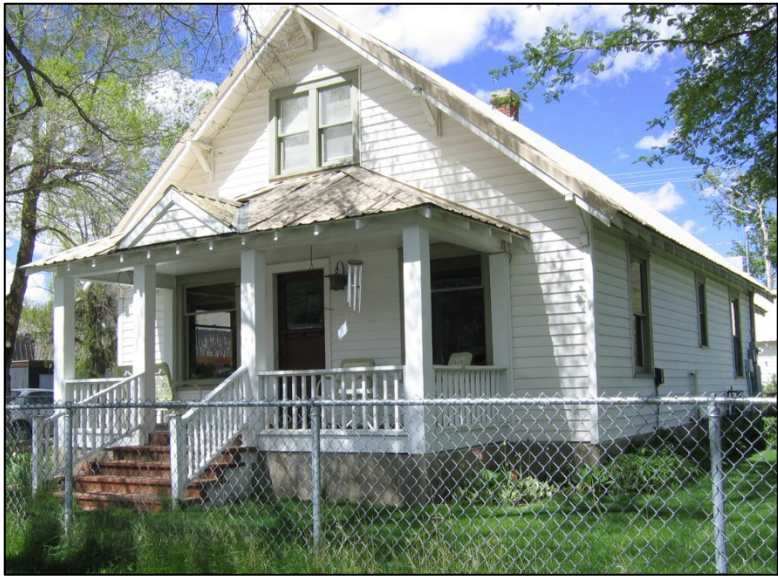
Figure 2: Existing Historic Home at 180 N Leadville
