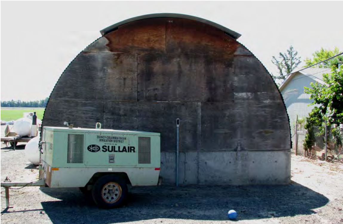
Figure 8: Building No. 1423 looking southeast at northwest elevation. Note the solid plywood wall where windows and clapboard had been. June 5, 2015. Reclamation digital photo by Kelsey Doncaster.
