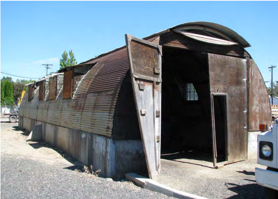
Figure 7: Building No. 1423 looking north at oblique view of southeast and rear elevations. Note the plywood double doors on the southeast end and plywood wall. June 5, 2015. Reclamation digital photo by Kelsey Doncaster.
