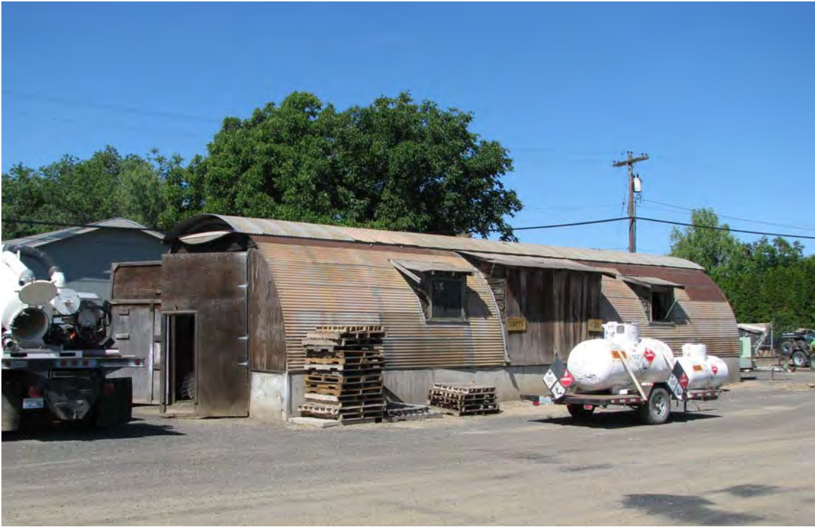
Figure 6: Building No. 1423 looking west at oblique view of front and southeast elevations. Note that the Quonset Hut has been raised on a concrete foundation along with removal of the original side entrance with windows. June 5, 2015. Reclamation digital photo by Kelsey Doncaster.
