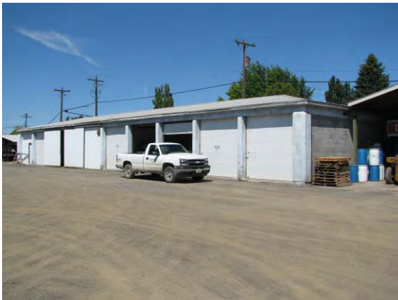
Note all original wood roll-up doors are replaced with vinyl, bay 1 & 5 are closed off and a sliding door over bay 3 & 4. Reclamation digital photo by Kelsey Doncaster. 6/5/2015. Oblique view of front and east elevations of Building No. 1454. 2015
