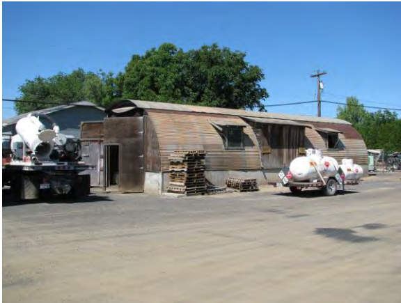
Note that the Quonset Hut has been raised on a concrete foundation along with removal of the original side entrance with windows. Reclamation digital photo by Kelsey Doncaster. 6/5/2015. Building No. 1423 looking west at oblique view of front and southeast elevations. 2015
