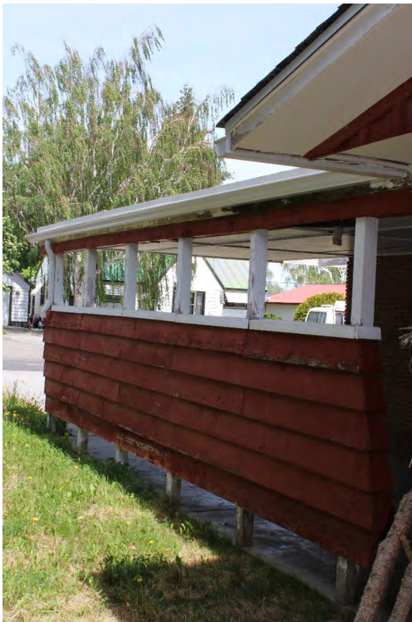
7. West Elevation showing horizontal lapped boards over posts on the carport, looking northeast.
