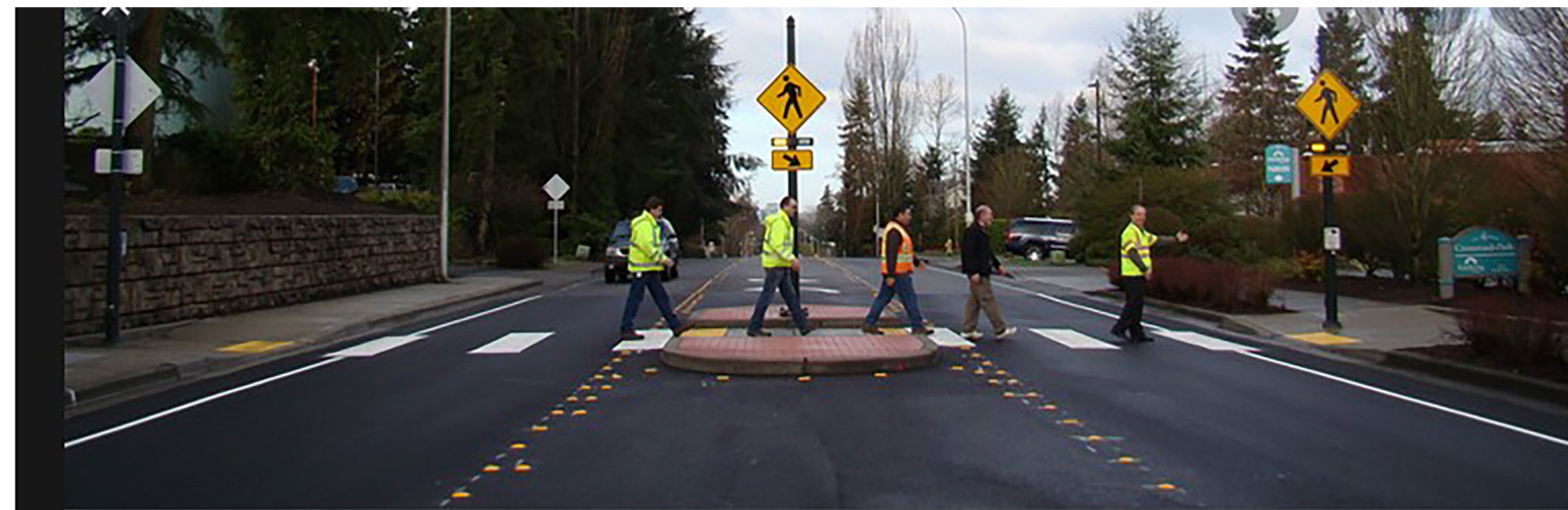
Median Rapid Flashing Beacon
