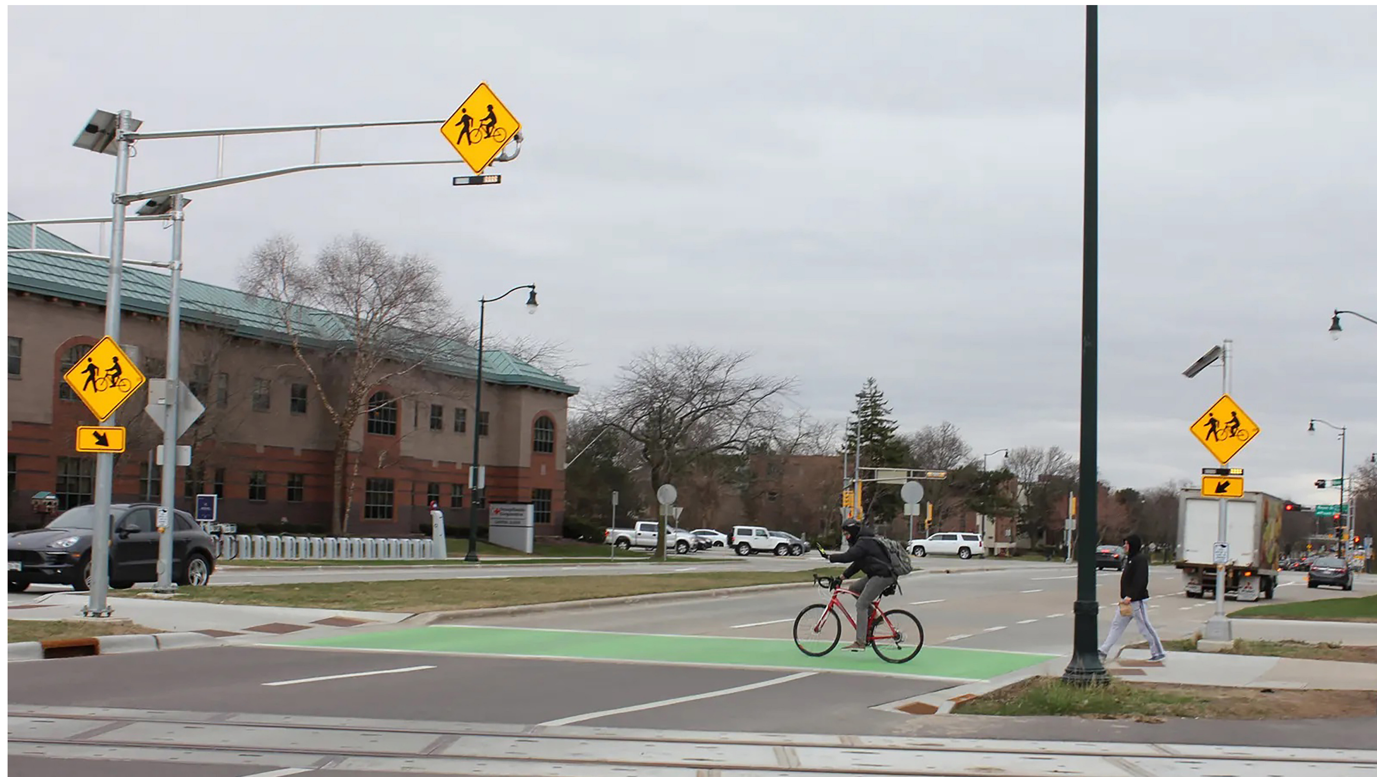
Overhead Rapid Flashing Beacon
