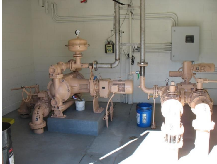
Figure 3-20. Biosolids transfer pump room
