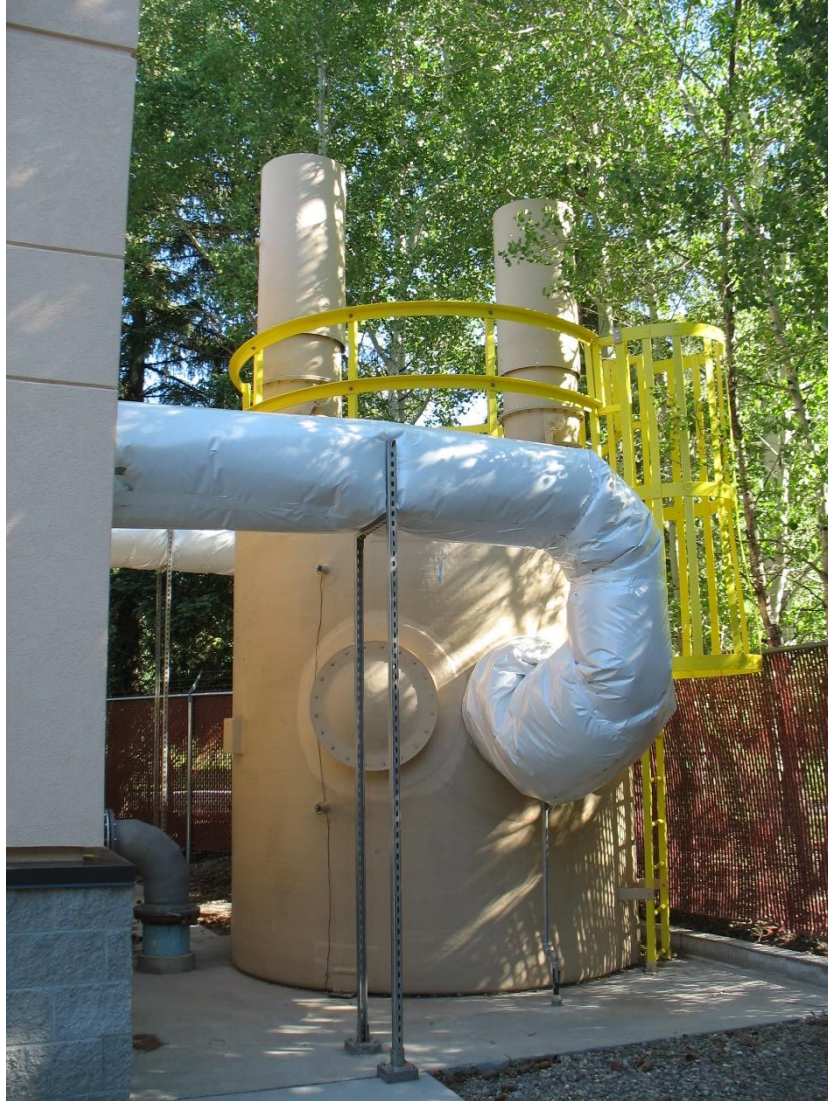
Figure 3-6. Carbon filter system for odor control
