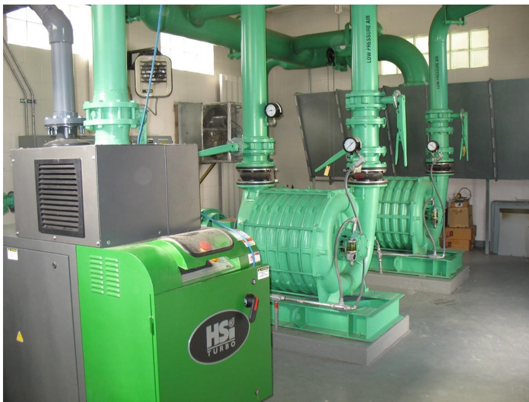
Figure 3-19. Digester blower room
