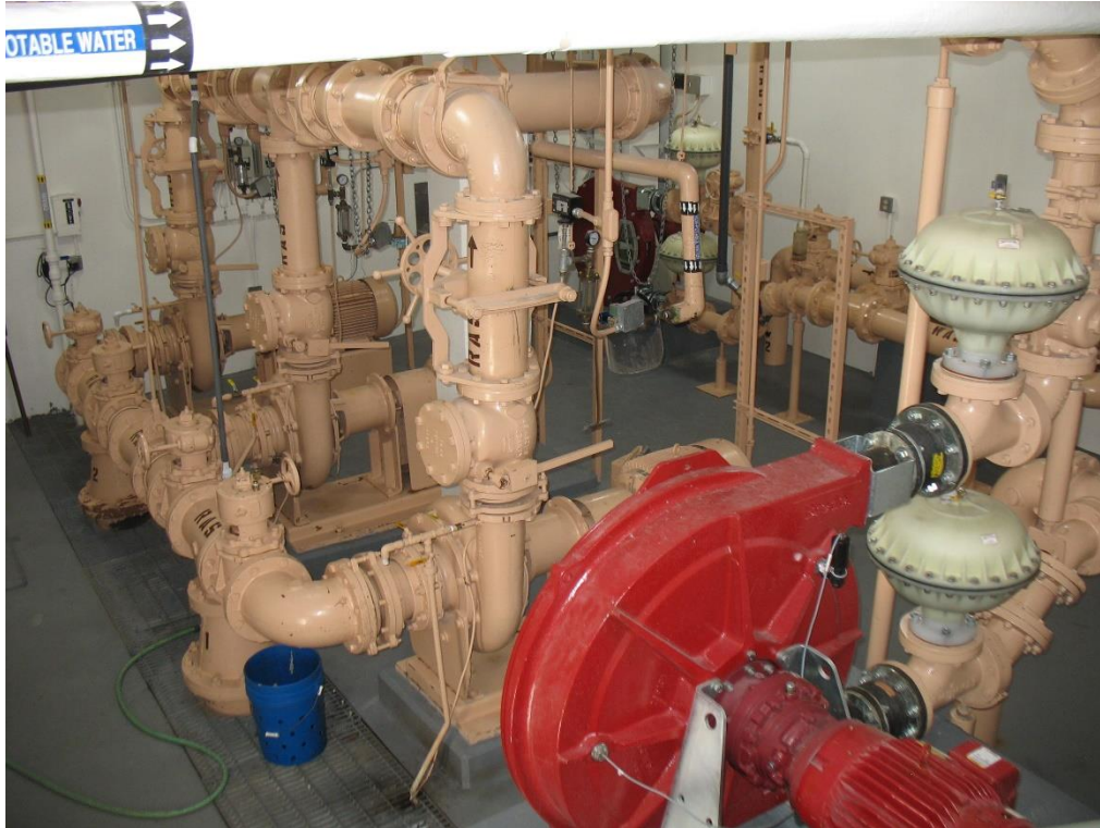
Figure 3-10. RAS and WAS pumping room
