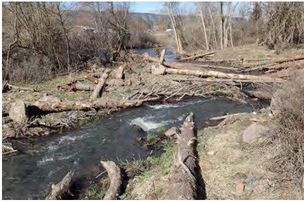
Side channel outlet, wood structure, and constructed riffle immediately after construction.
