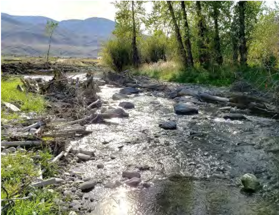
Constructed riffle in Subreach 3 one year after construction completion.
