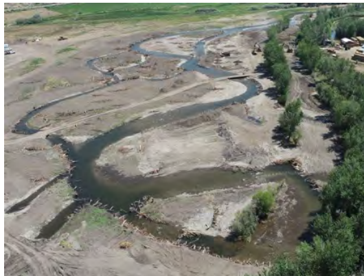
Subreach 1 Phase 1 under construction with mainstem recently activated.
