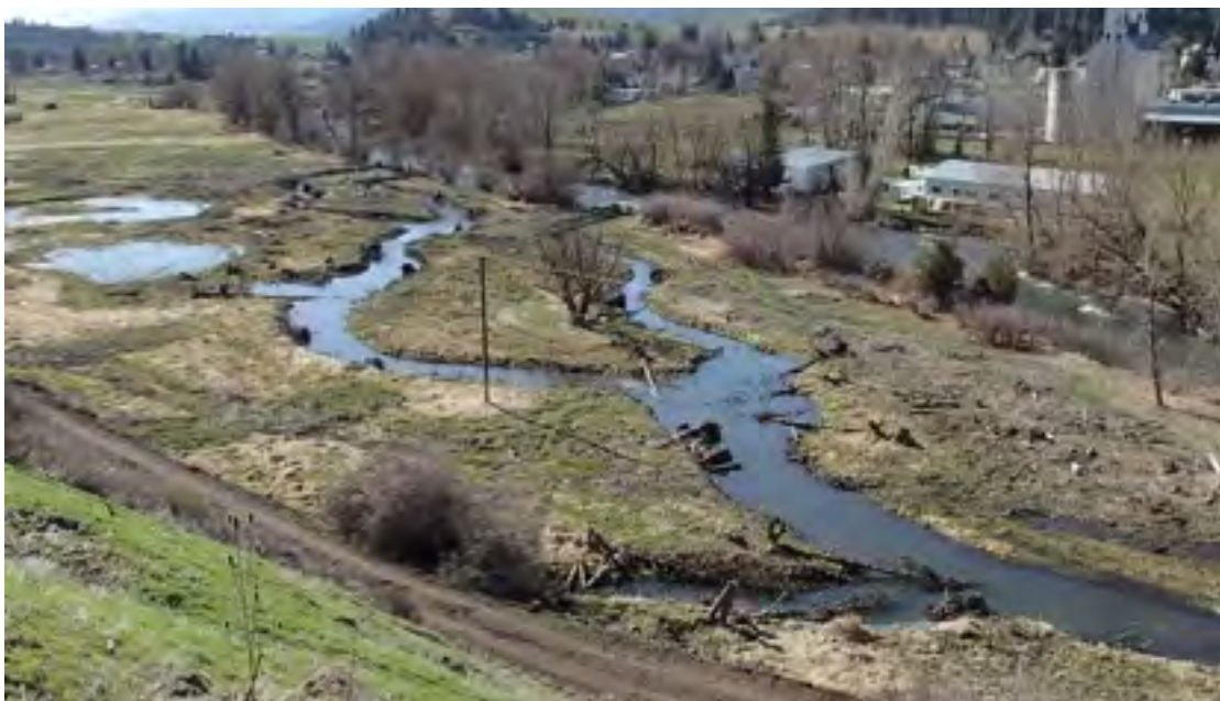
Oblique view of project area immediately after construction. Side channels and wetland/floodplain areas are activated.
