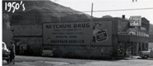
Windermere Real Estate Office
