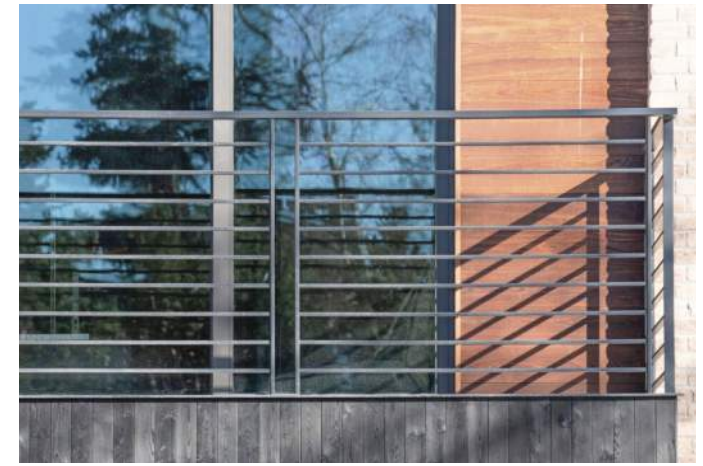
STEEL GUARD RAILINGS - galvanized and painted with WOOD TOP RAIL.
