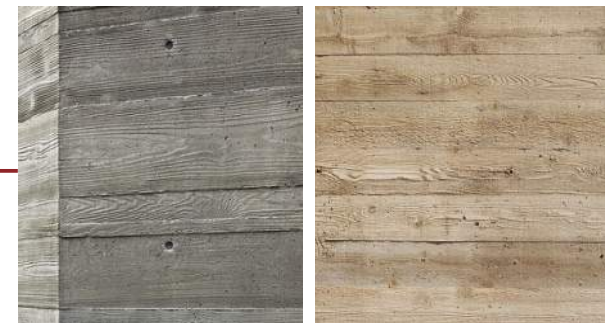
BOARD-FORMED CONCRETE - cast-in-place and stained.
