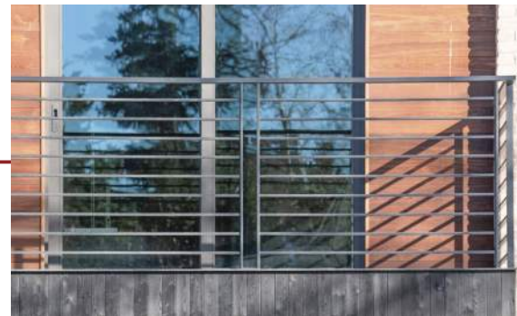
STEEL GUARD RAILINGS - galvanized and painted with Wood Top Rail.
