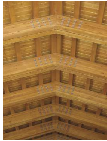
HEAVY TIMBER GLULAM BEAMS, RAFTERS AND COLUMNS with painted galvanized structural steel knife-plate connections. Fasteners to be recessed galvanized steel or stainless steel. Clear heart Western Red Cedar heavy timber purlins and T&G decking with resawn finish. Wood clear coat stain.
