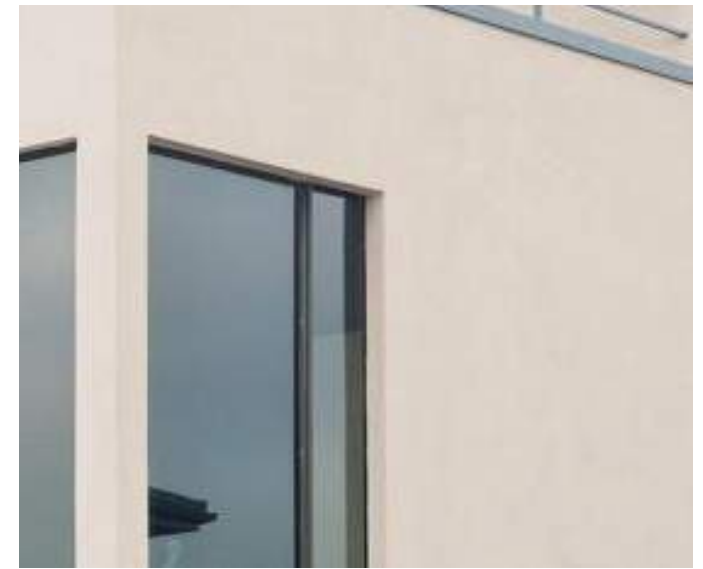
CEMENT PLASTER - 3-coat system, hard-troweled finish with 100% acrylic topcoat finish.
