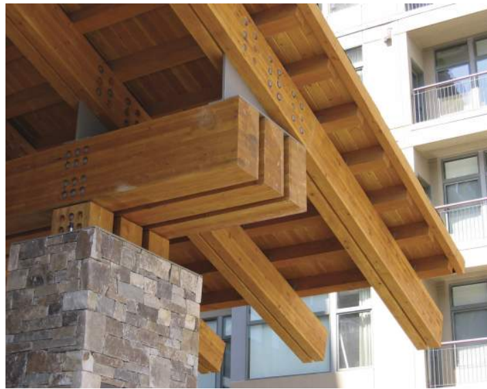
HEAVY TIMBER GLULAM BEAMS, RAFTERS AND COLUMNS with painted galvanized structural steel knife-plate connections. Fasteners to be recessed galvanized steel or stainless steel. Clear heart Western Red Cedar heavy timber purlins and T&G decking with resawn finish. Wood clear coat stain.
