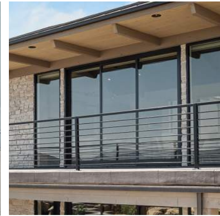
ALUMINUM WINDOWS AND DOORS - powder coated extruded aluminum with Low "E" insulated glass. Basis of Design: Vistaluxe Collection AL Line - Kolbe Windows and Doors. Basis of Design: Reynaers CP155LS Monorail System.
