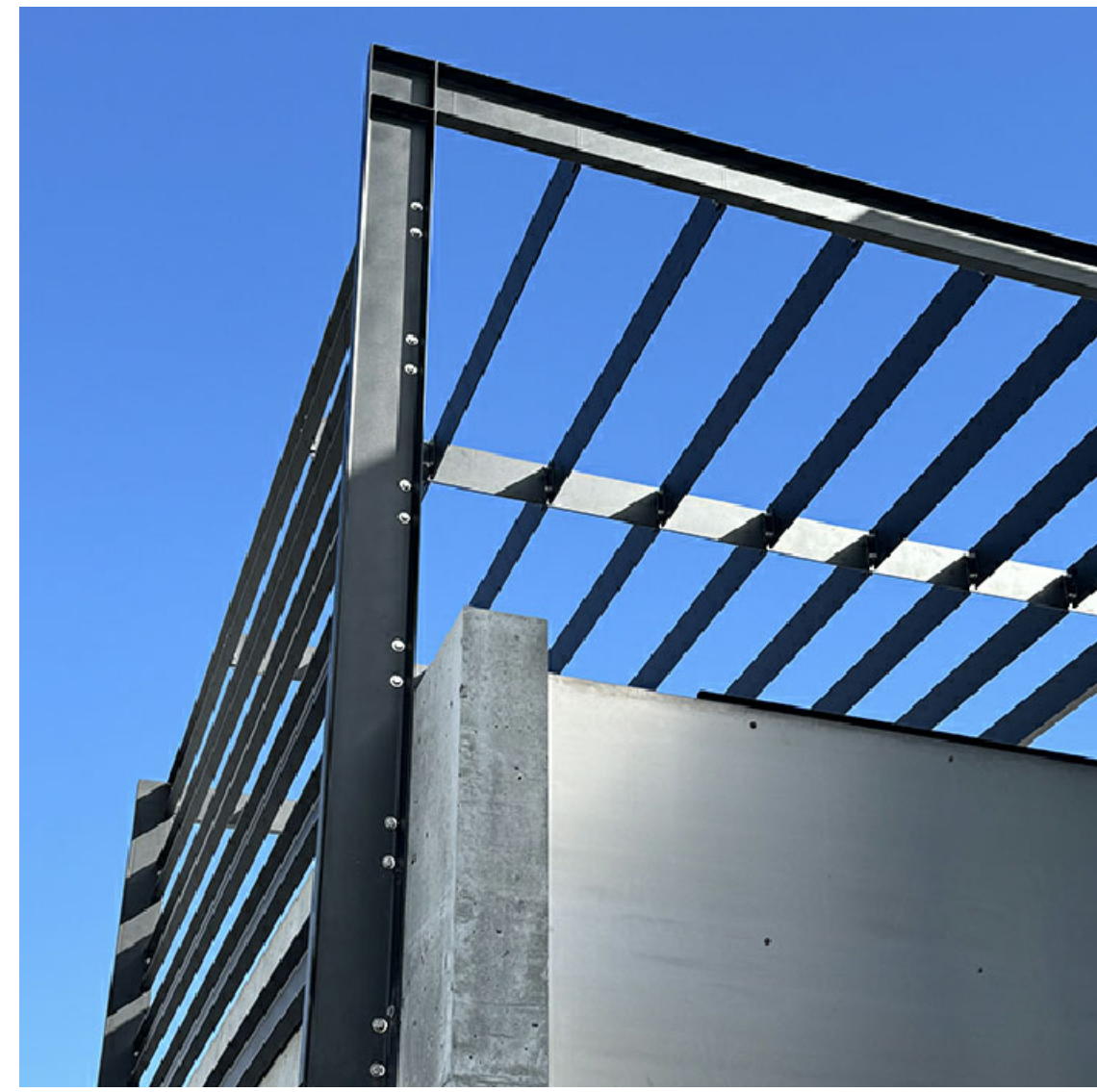
ROOF TOP TERRACE TRELLIS
