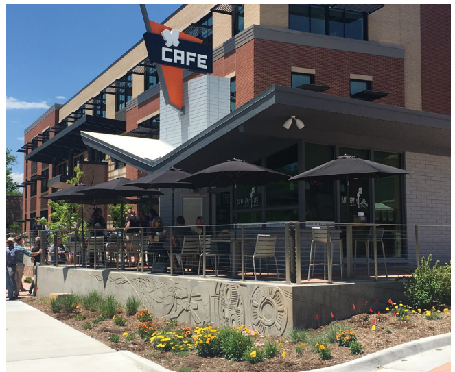
Logan Simpson assisted with the development of the award-winning Utility Administration building which preserved the historic “Butterfly Building”, incorporating it into the overall site design, and repurposing it for a quaint, and very popular, walk up café.
