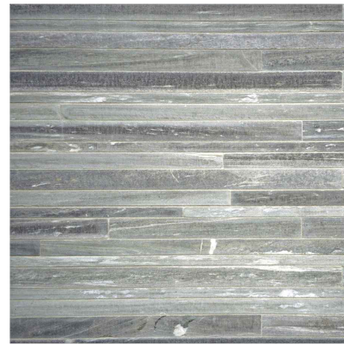
3) Stone Cladding At exterior walls
