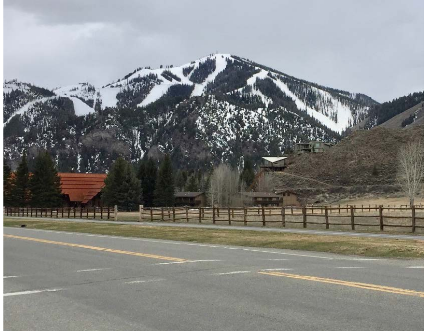
Figure 4: Existing Non-conforming Buildings Visible on Hillside
