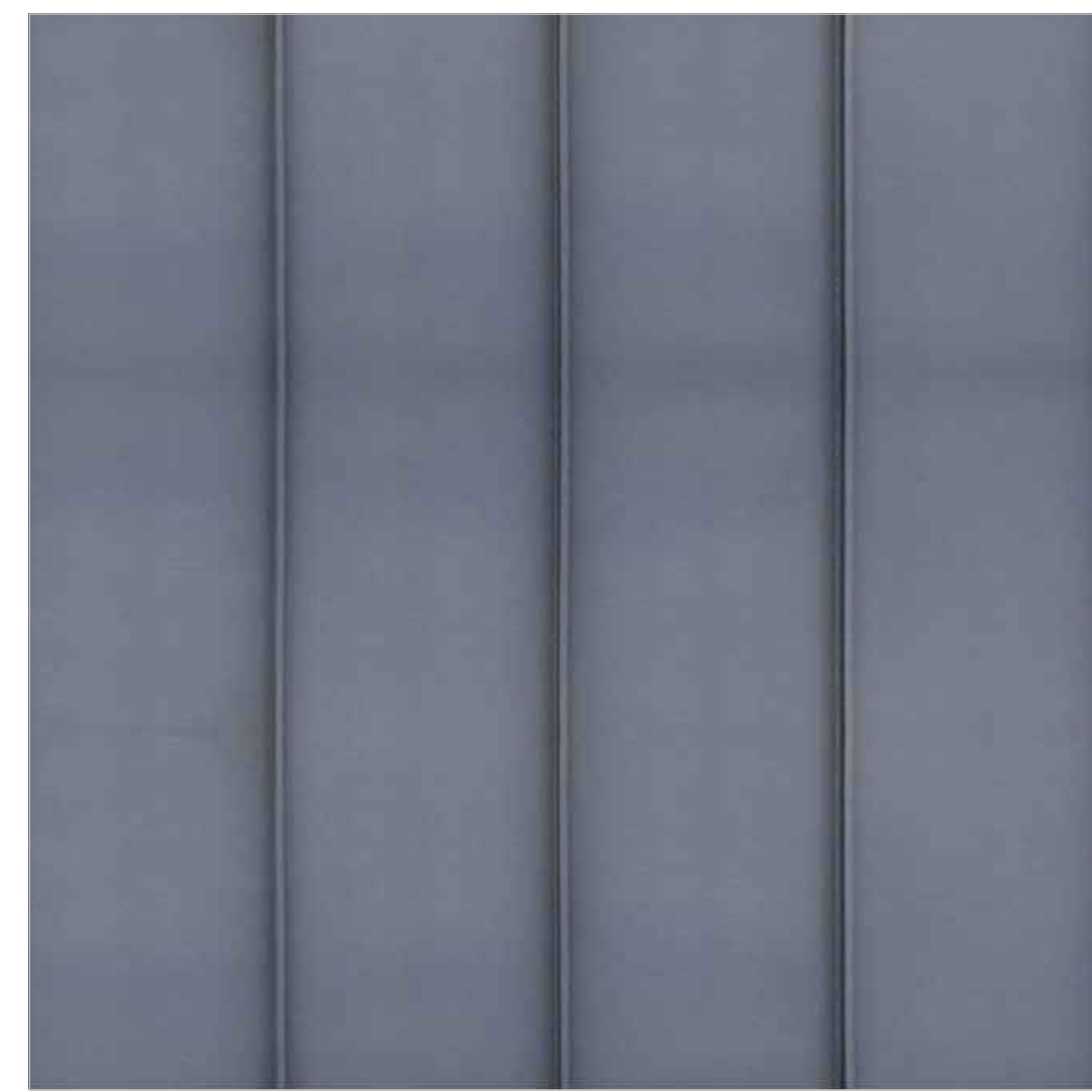
6) Zinc At chimneys & parapet caps
