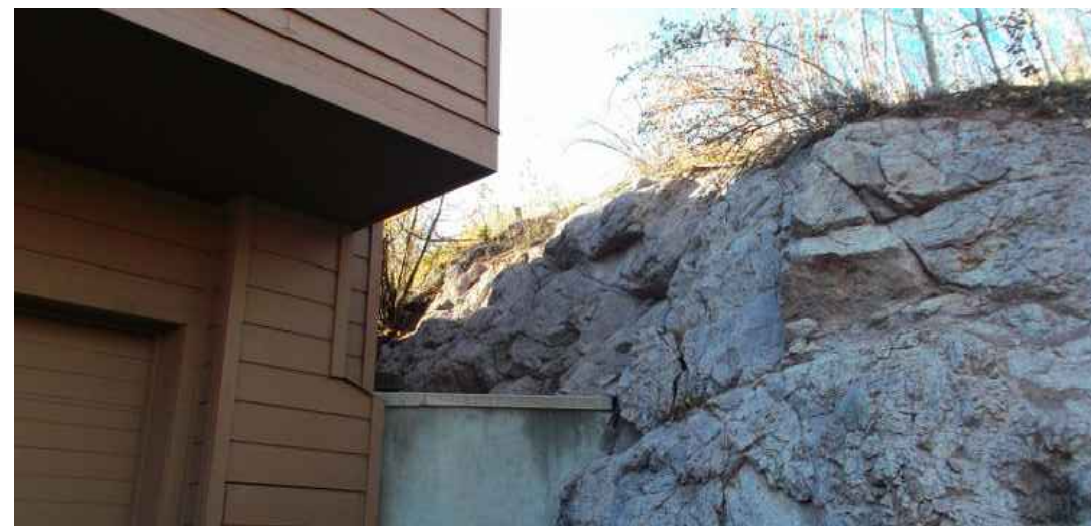
2) View from driveway
