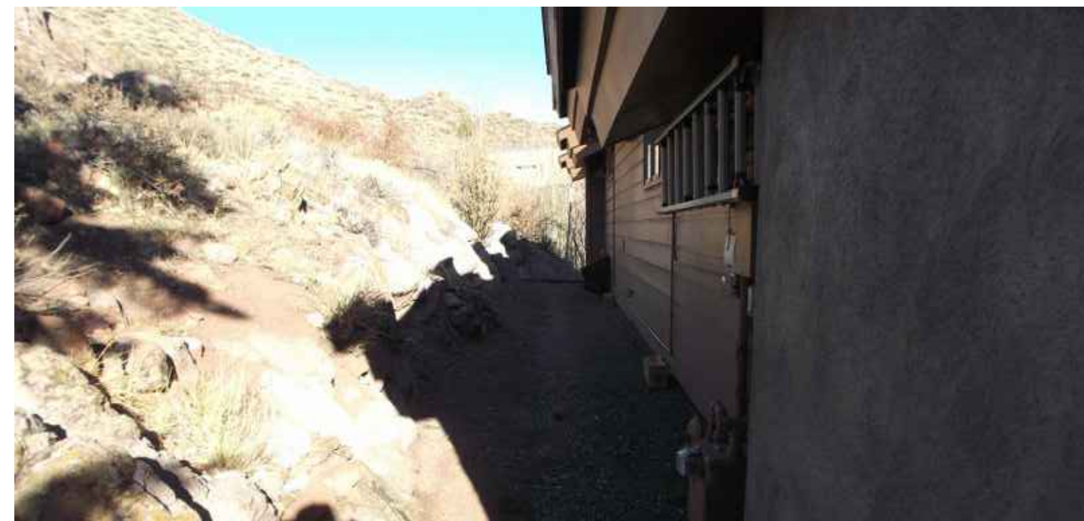
1) View at back of existing house
