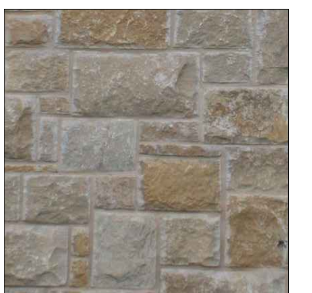
Typical Stone Veneer Light limestone, wide grout joints
