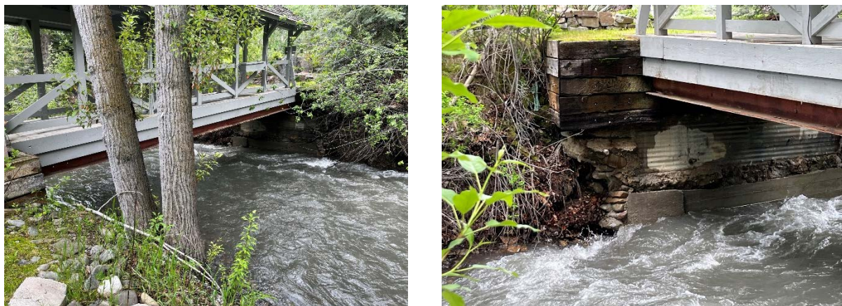
Figure 11 – Pedestrian Bridge & Abutment
