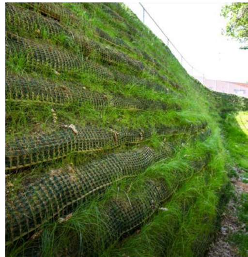
Figure 9 - Wrapped-Face Geosynthetic Reinforced Slope, Installed
