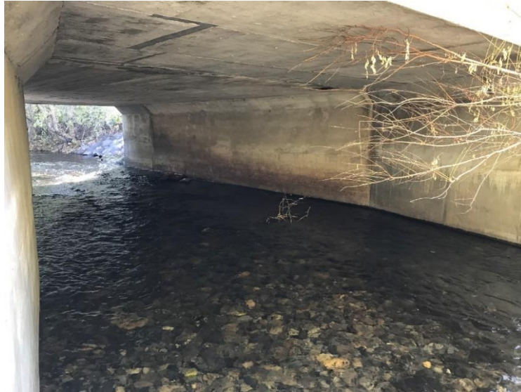
Photo 4. Looking upstream under SH-75 Bridge over Trail Creek on October 8, 2019.
