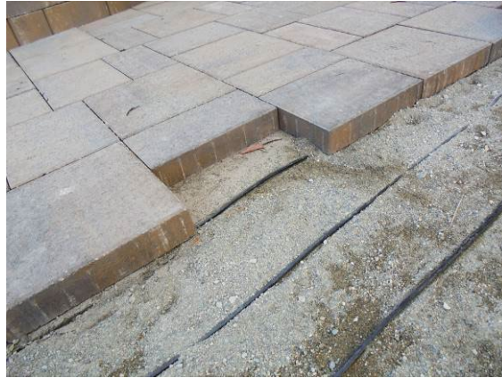
Pavers with radiant snowmelt system integrated.
