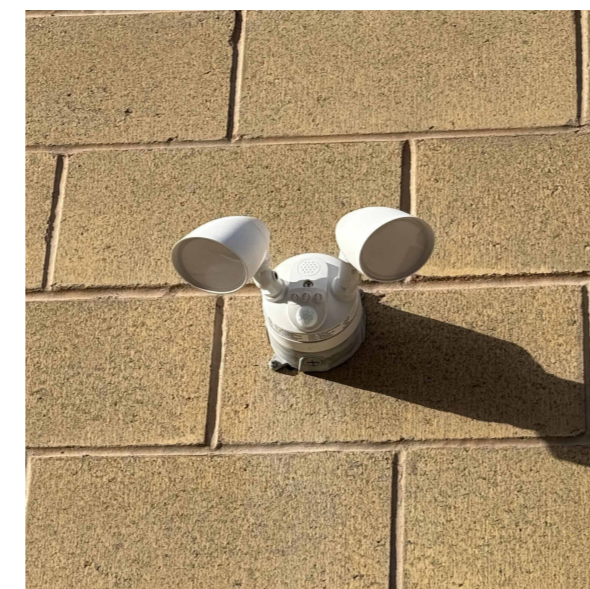
E4 FLOOD LIGHT - MOTION ACTIVATED SHALL BE ANGLED SO THAT NO LIGHT ESCAPES ABOVE A 25° ANGLE MEASURED FROM A VERTICAL LINE EXTENDING FROM THE CENTER OF THE FIXTURE TO THE GROUND 2700K 20W, 1960 lm ± *COLOR TEMPERATURE TO BE VERIFIED BY OWNER & FIXTURE MODIFIED / REPLACED AS NECESSARY TO MEET CITY OF KETCHUM LIGHTING STANDARDS
