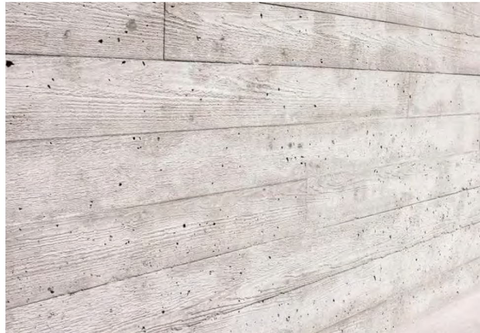
board formed concrete
