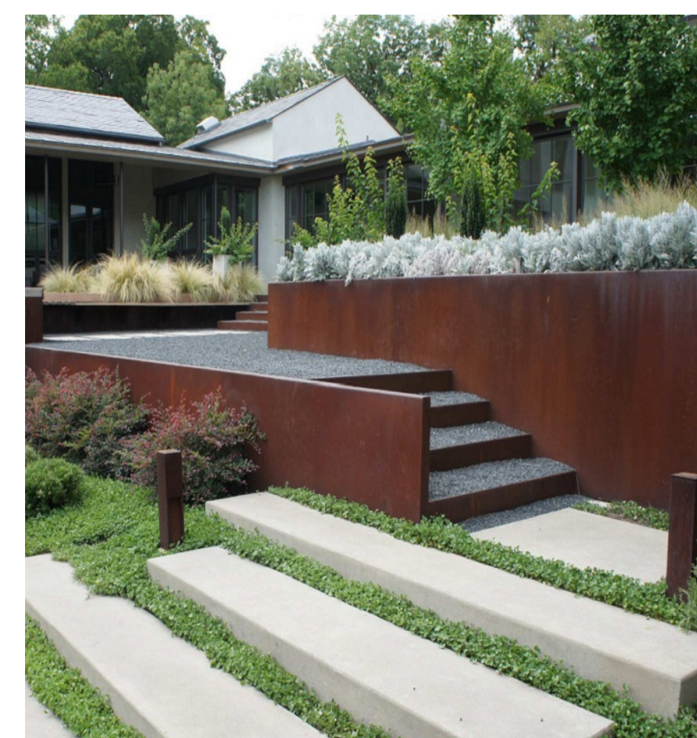
CONCRETE W/ STEEL PLANTERS AS RETAINING WALLS
