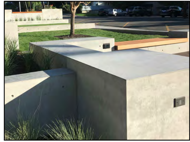
ARCHITECTURAL CONCRETE SITE WALLS
