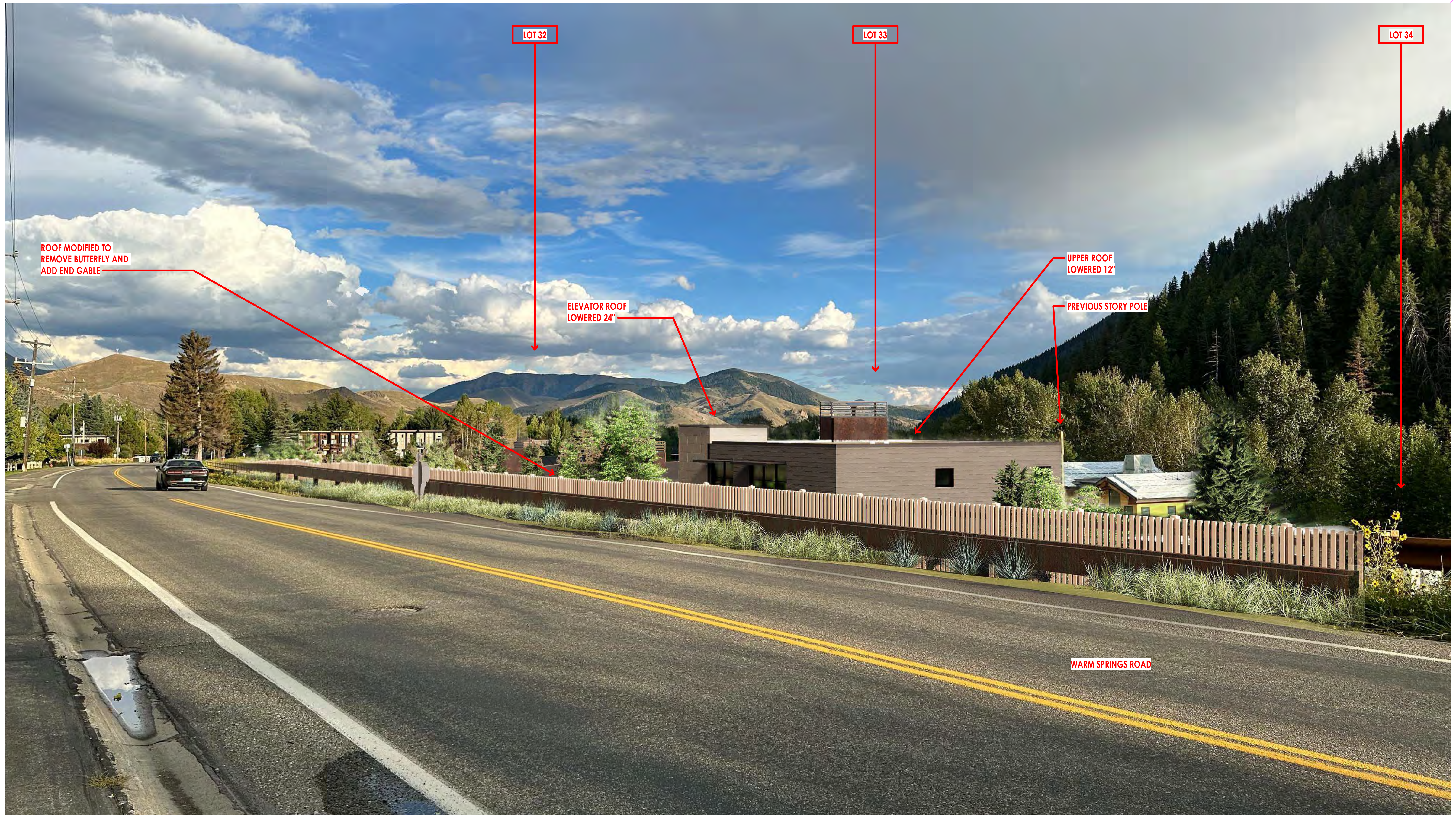
WARM SPRINGS ROAD LOOKING EAST
