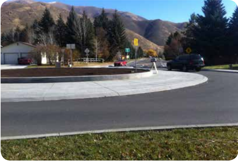
Roundabout at Woodside Boulevard and Fox Acres calms traffic while keeping traffic moving.
