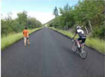
Road sealed with "chip sandwich"
