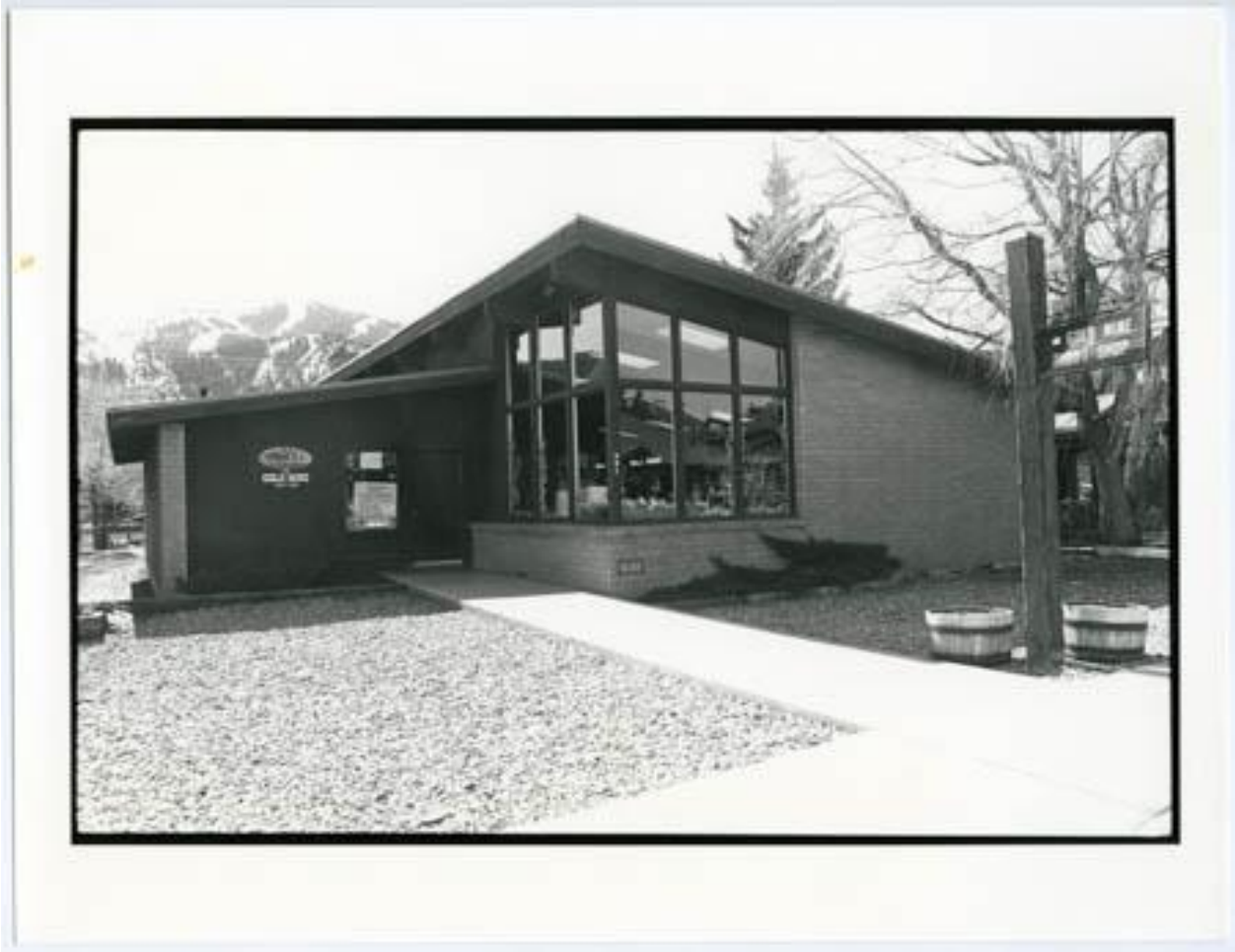
The Community Library / Gold Mine Building, circa 1957
