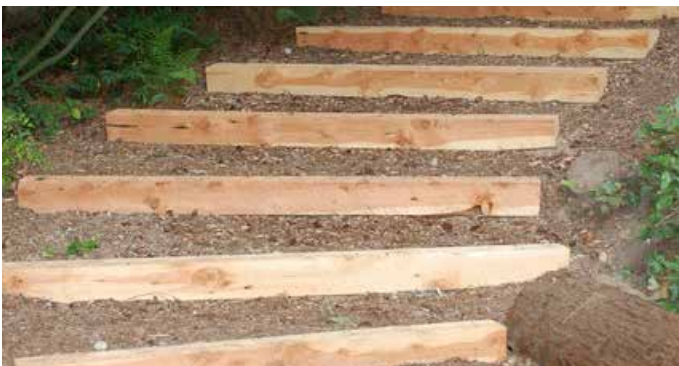
Natural timber steps set into the hillside with steel braces
