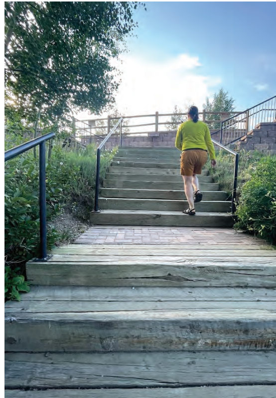
Existing stair conditions. Left: Steps made of local wood and connected by brick paved landings. Gravel paths below. Right: Climbing existing steps heading toward the parking lot.
