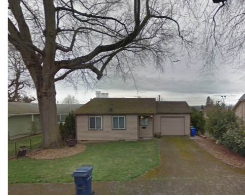
3 NE SARATOGA RESIDENCE
