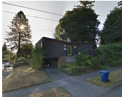
6 NE 27TH RESIDENCE
