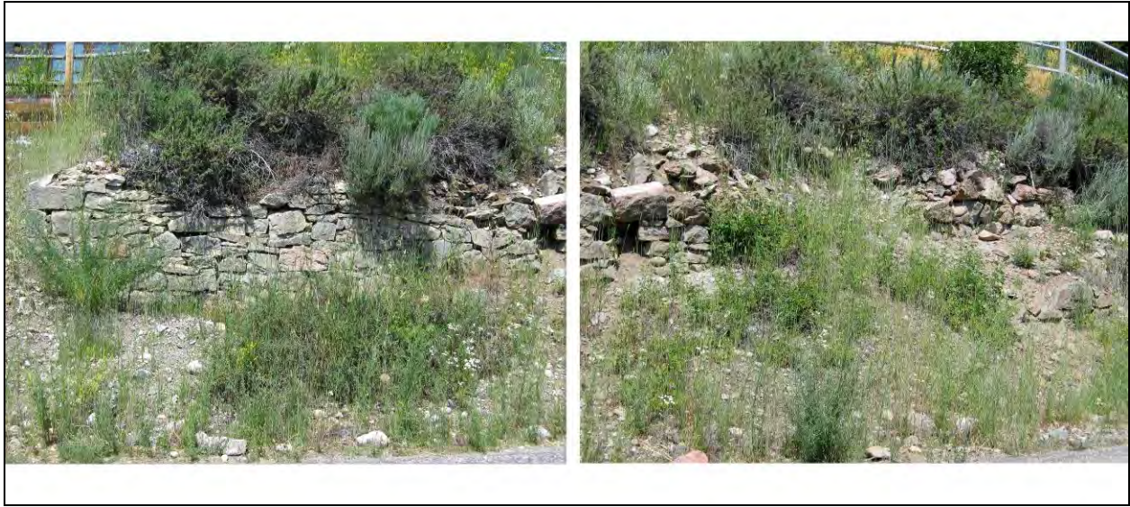
Figure 17a. View of east facing wall along Exhibition Boulevard looking west. Digital Image WS 37 # 20.
