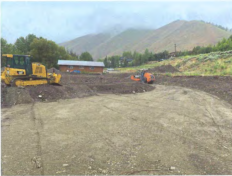
Imported sand and gravel placed in 10" loose lifts, watered and compacted with multiple passes of a vibrating smooth drum roller as structural fill. 29Jun20
