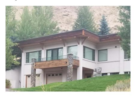
Figure 2 – Shed Roof Design at 104 Sage Road
