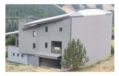
Figure 3 – Blocking Wall Design at 100 Sage Road (Note that doors are reinforced, windows are small, recessed, or 10-ft. above grade.)
