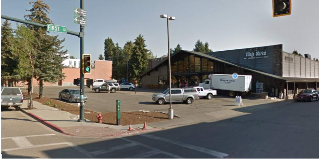
Figure 9. Large Access and Lack of ADA/PROWAG Compliant Facilities at 1 st Street
