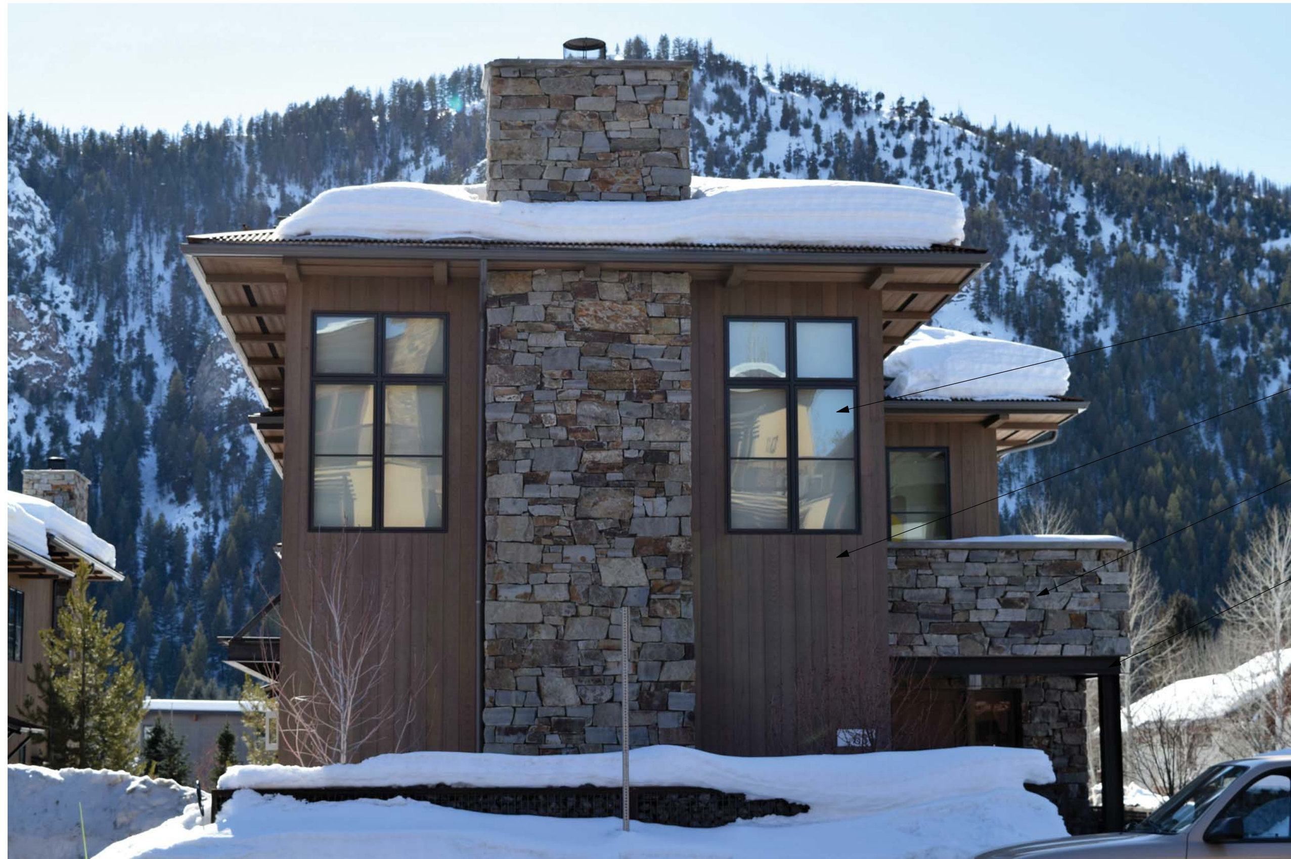
EXISTING CROSSBUCK TOWNHOMES 1 MATERIAL REFERENCE PHOTO
