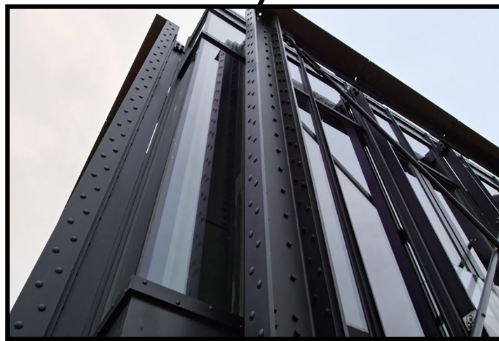
PAINTED METAL FACADE
