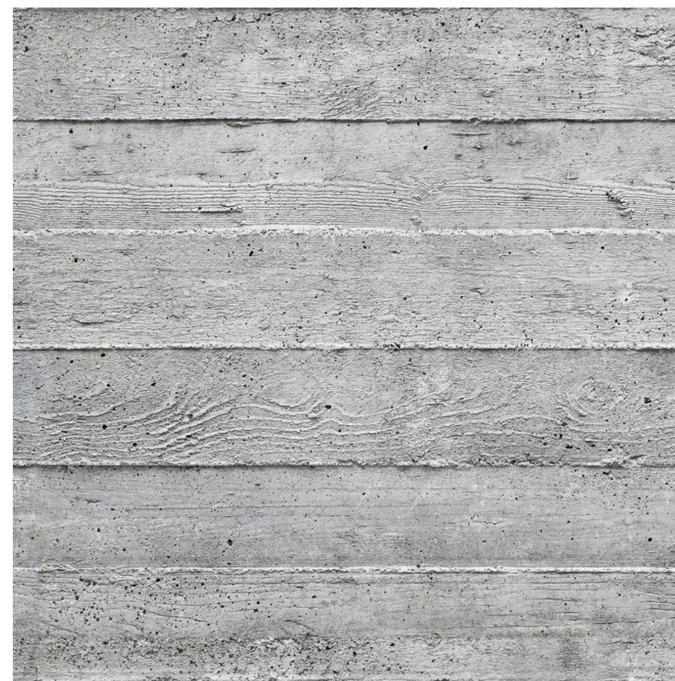
BOARD FORMED FINISH CONCRETE
