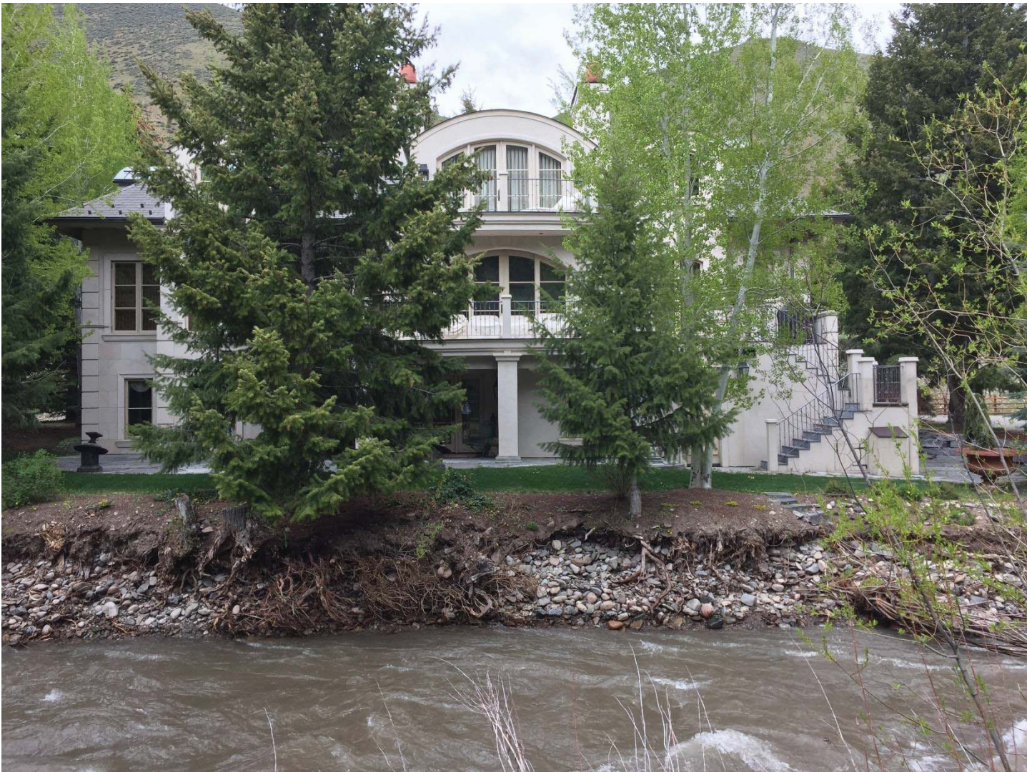
Site photos, May 2017
