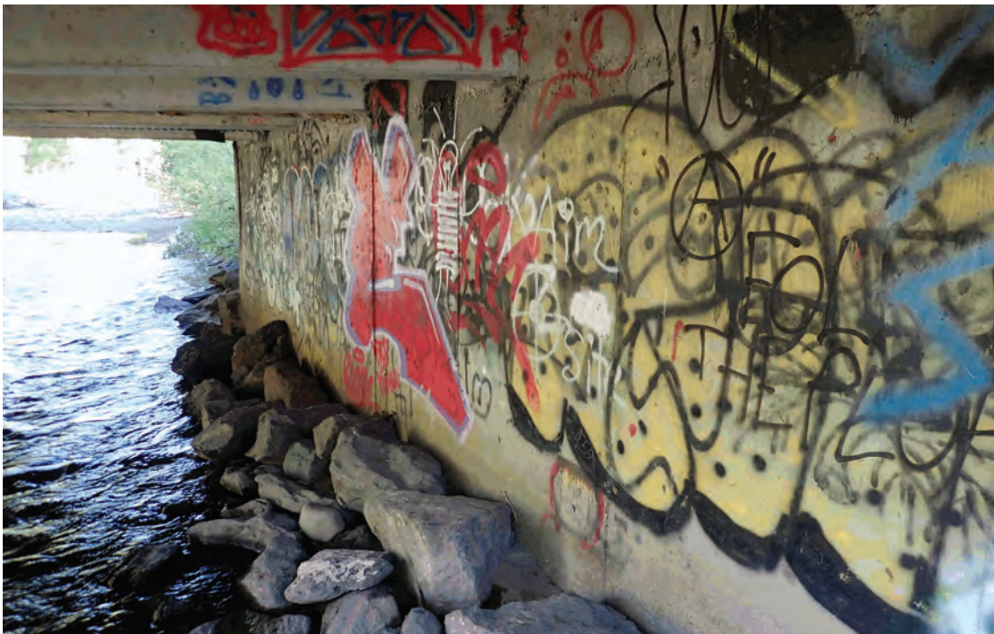
East abutment looking northeast.
