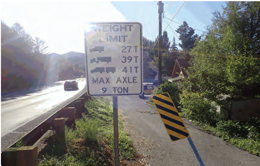
Weight limit sign at west approach looking east.
