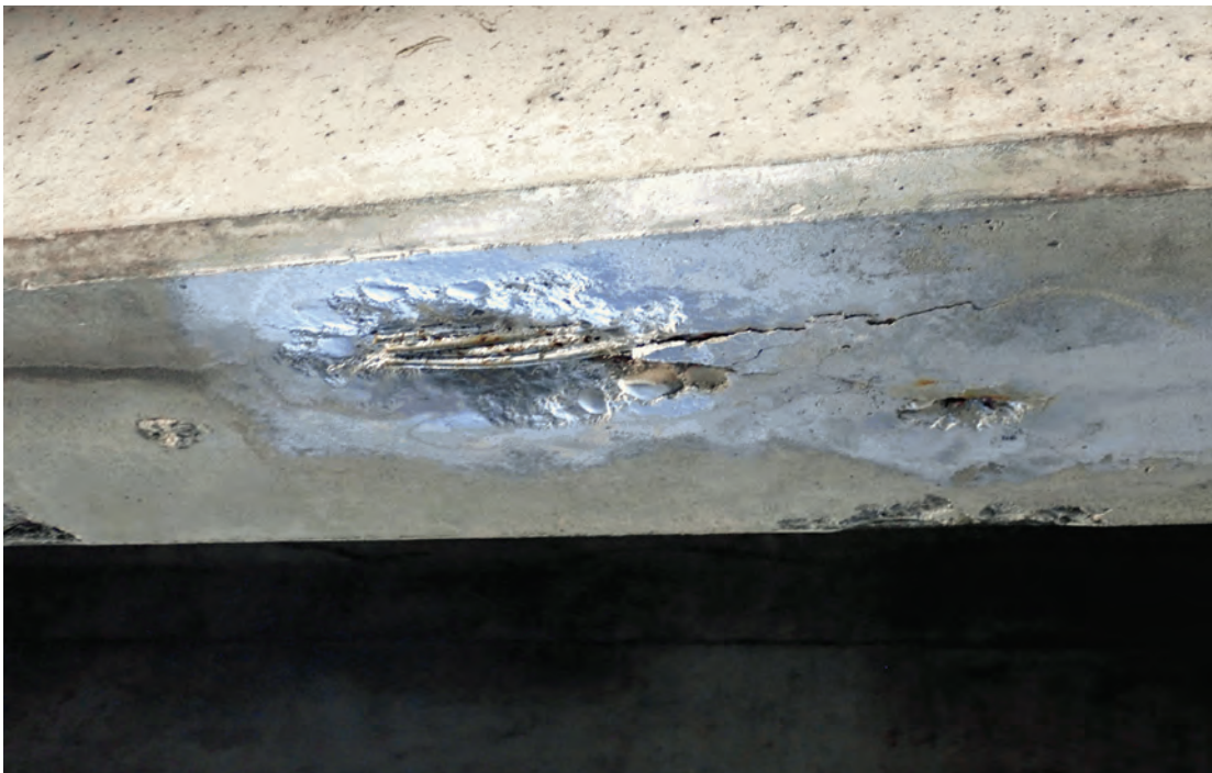
Exposed prestressing looking north.
