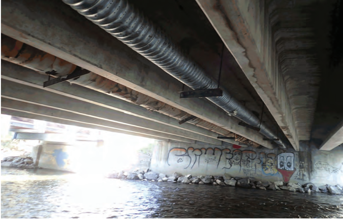
Underside and west abutment looking southwest.
