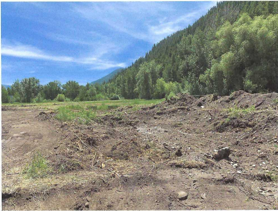
Organics, debris and disturbed soils to be removed prior to placing structural fill to match adjacent existing grade. 26Jun20
