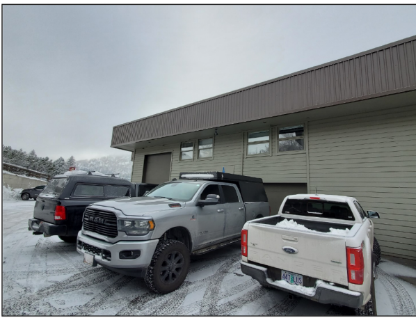
Exterior View (Front)
