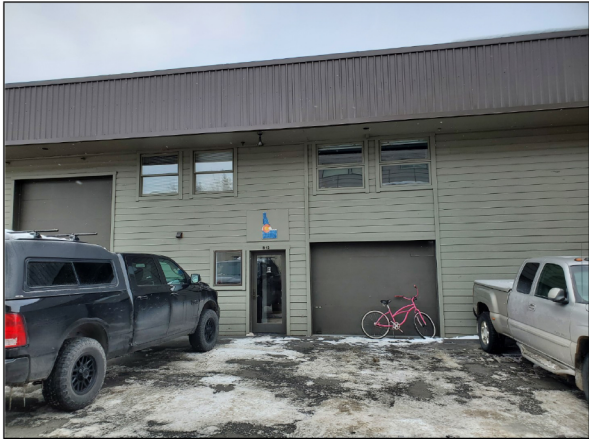
Front View (subject on 1 st & 2 nd Levels)
