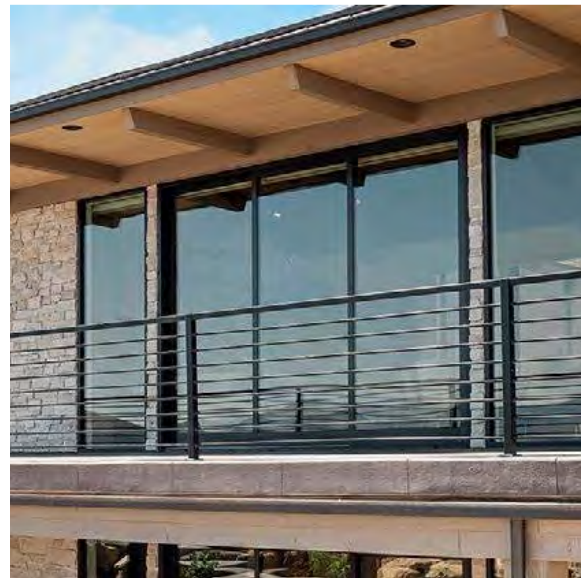
ALUMINUM WINDOWS AND DOORS - extruded aluminum with Low "E" insulated glass. Basis of Design: Vistaluxe Collection AL Line - Kolbe Windows and Doors. Basis of Design: Reynaers CP155LS Monorail System. Basis of Design: Sherwin-Williams Fluoropon 70% PVDF Coating System
