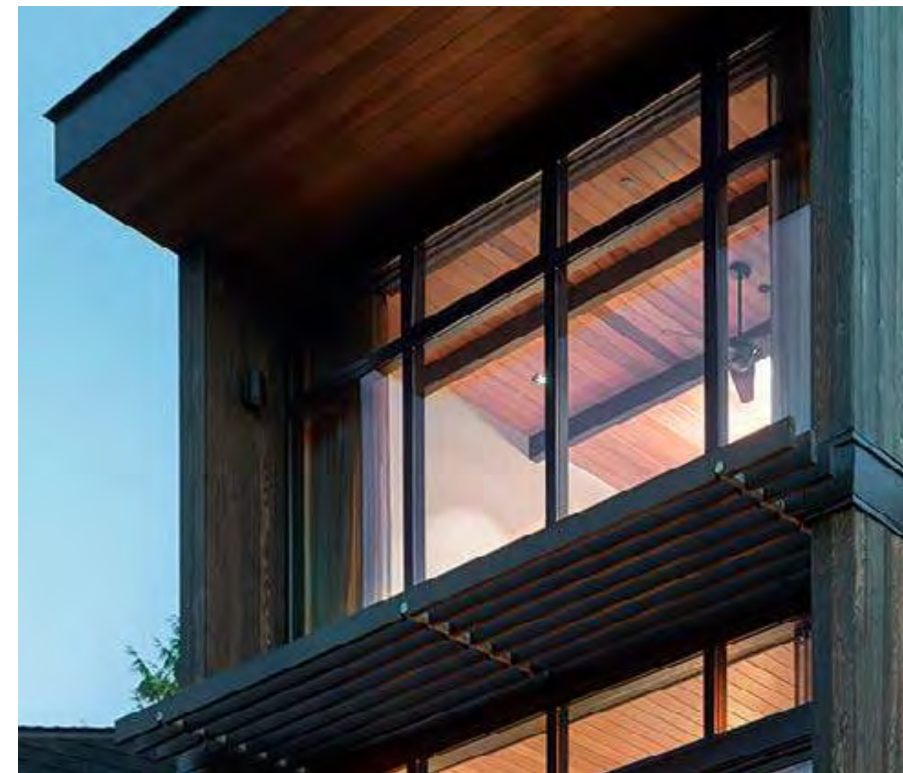
ALUMINUM WINDOWS AND DOORS - extruded aluminum with Low "E" insulated glass. Basis of Design: Vistaluxe Collection AL Line - Kolbe Windows and Doors. Basis of Design: Reynaers CP155LS Monorail System. Basis of Design: Sherwin-Williams Fluoropon 70% PVDF Coating System
