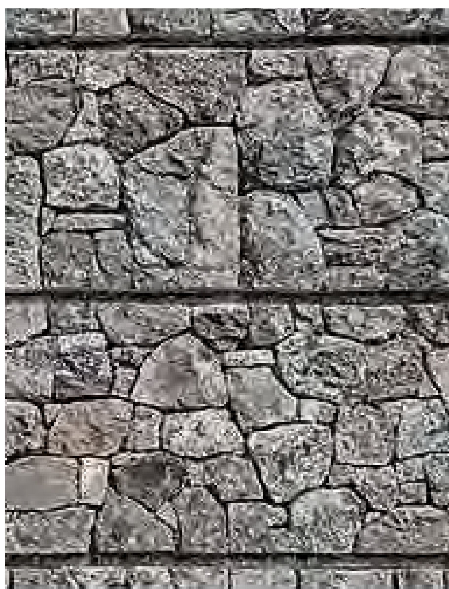
STONE VENEER - Natural stone with stainless steel masonry anchor system. Montana Moss Rock or Basalt
