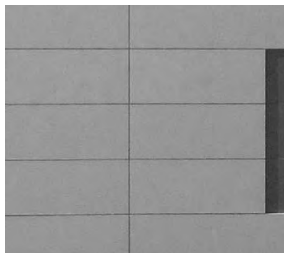
METAL PANELS - 24" X 60" with PVDF finish. Basis of Design: EN-V Architectural Metal Panel System.
