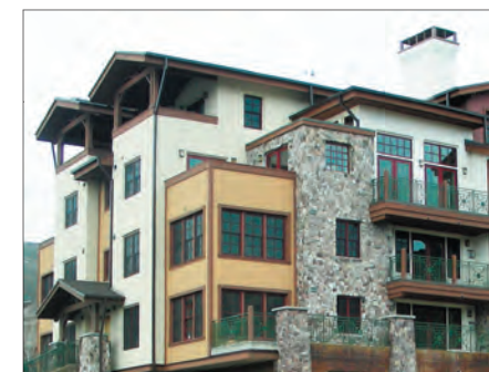
A flat roof may be used as an accent to break up the perceived mass of the overall building
