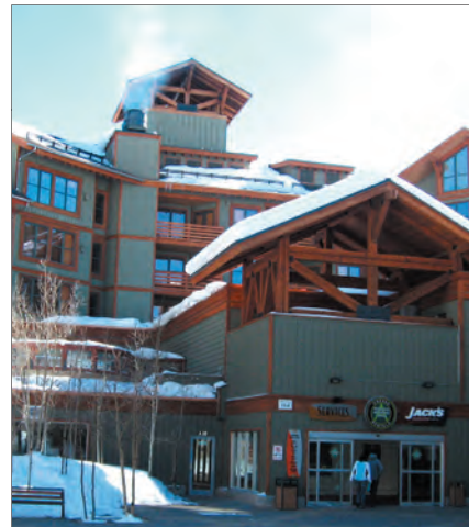
A secondary façade may be offset for improved views and/or solar access.
