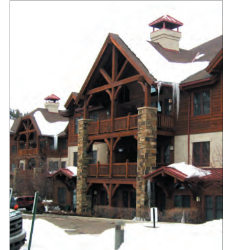
Design sloping roofs to shed onto other roof forms or onto snow storage areas on site.
