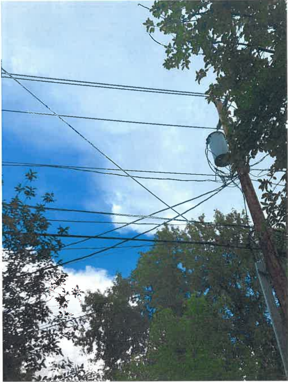
VIEW FROM LOT AT 760 WASHINGTON AVE
