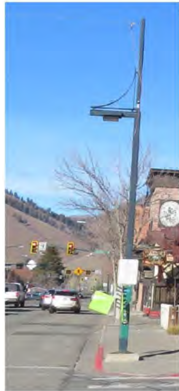
Approximate location of existing streetlight to be re-lamped Fixture height: ±16'-6"
